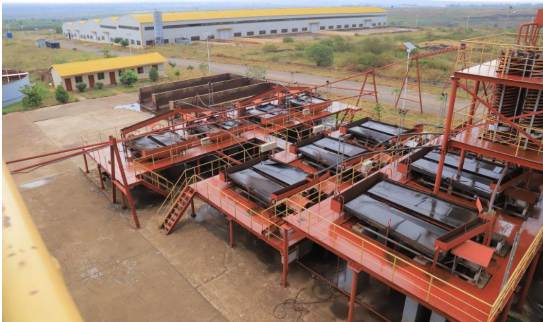
A section of the Phosphate plant in Tororo
